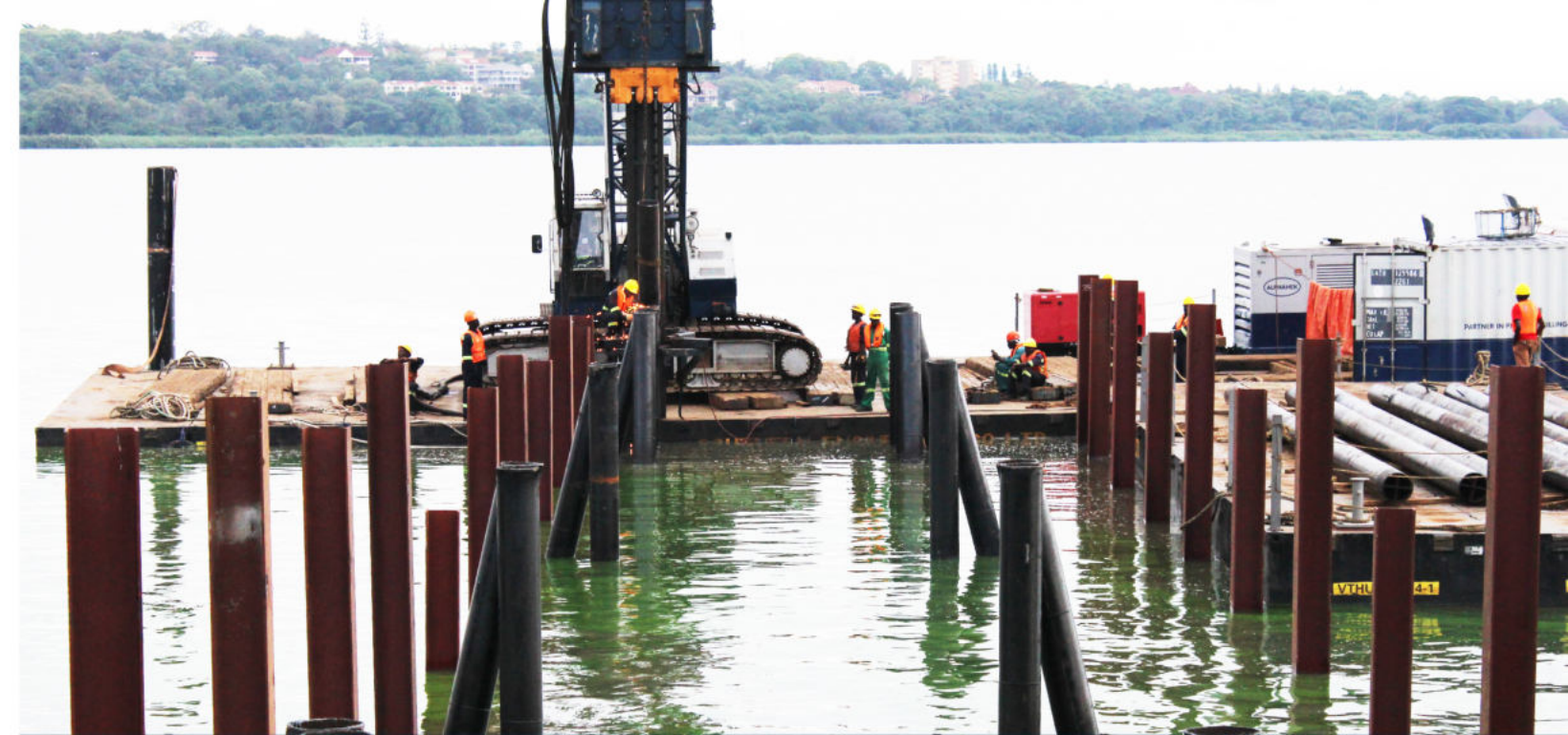
PILING WORKS - KISUMU OIL JETTY, KENYA
