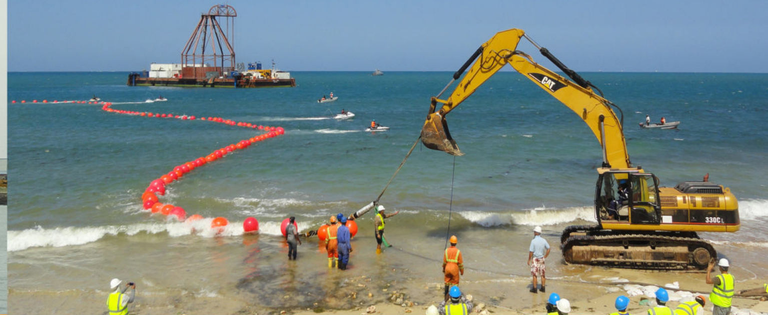
FIBRE OPTIC CABLE LAYING ZANZIBAR TO DAR ES SALAAM
