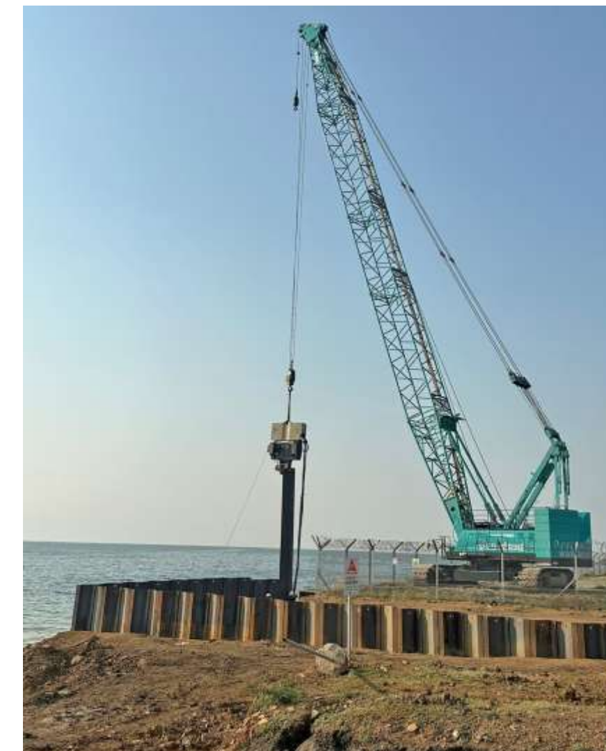
SECO Marine (U) Ltd begins the installation of Sheet piles at Kingfisher Development Area, Southeast of Lake Albert, Uganda
